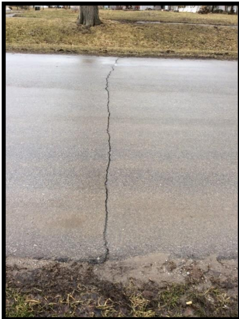
Transverse Cracking
