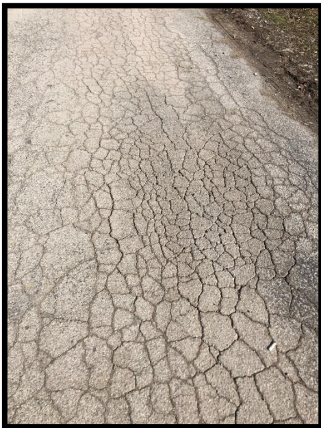
Alligator Cracking
